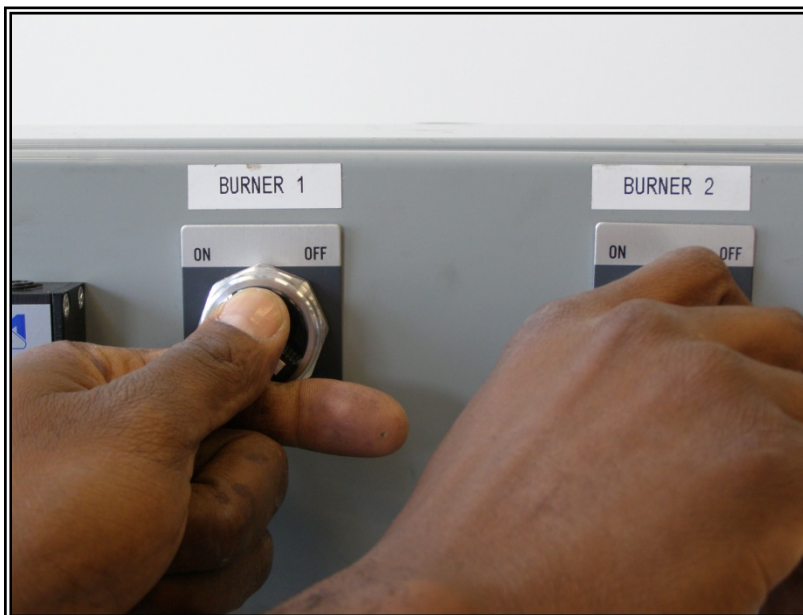
Figure 3. Step 9 Turn burner switches to "ON" position.
