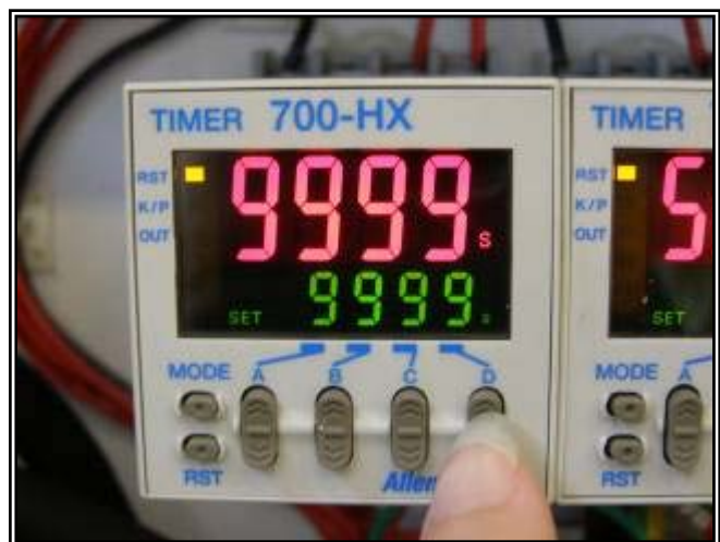
Figure 46. Step 5 Timer set to maximum time
