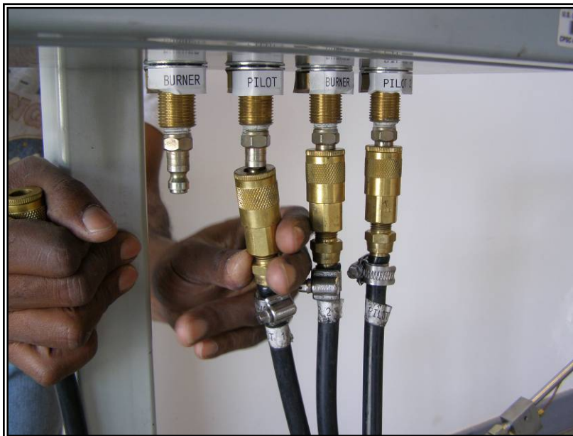
Figure 10. Step 3 Connect hoses to control box.
