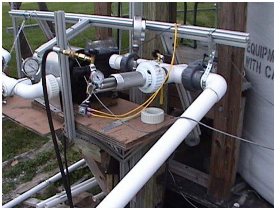
Figure 2 Pump and air vent installation (Source: Mark Eilbert of CPSC)
